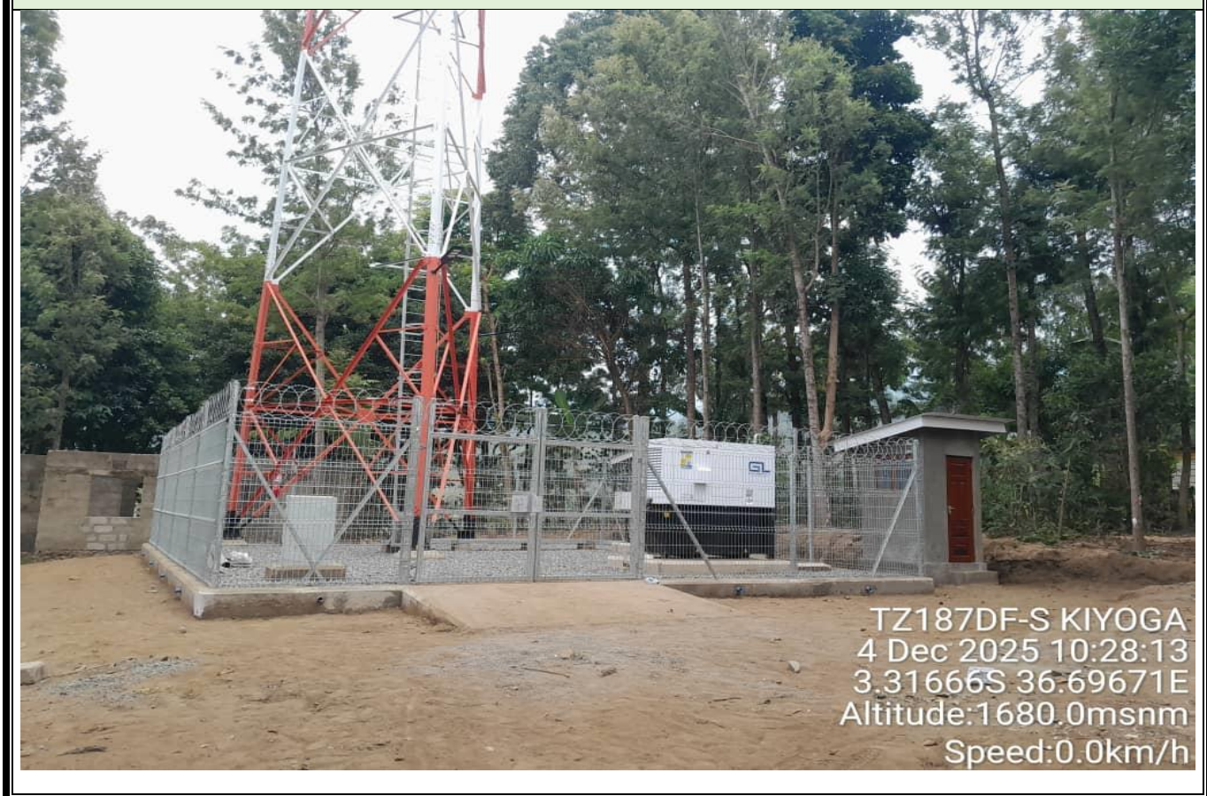
FRONT VIEW OF SITE WITH SIGNAGE ON GATE (1 PHOTO)
