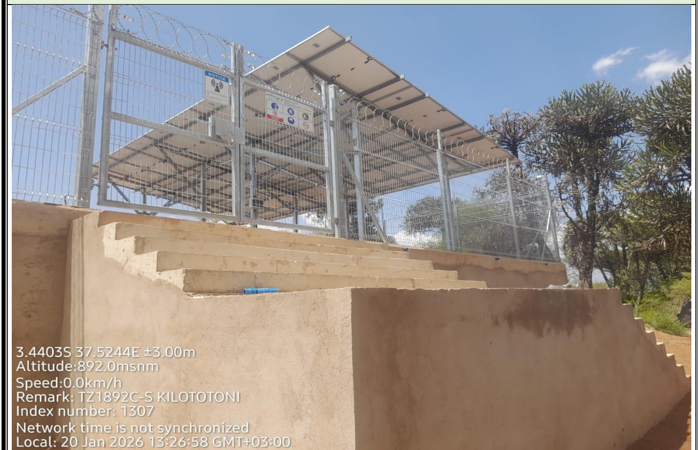
FRONT VIEW OF SITE WITH SIGNAGE ON GATE (1 PHOTO)
