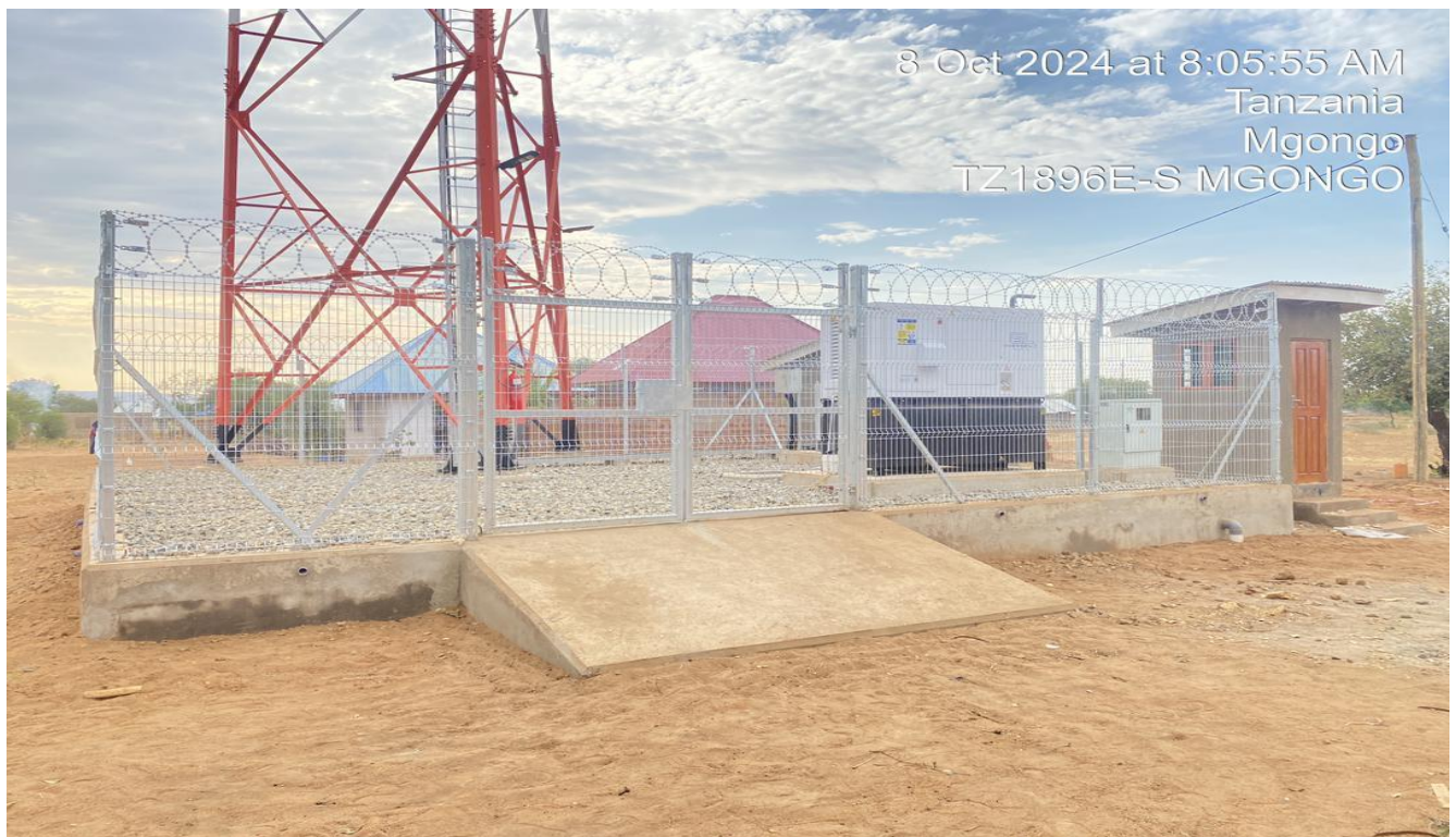
FRONT VIEW OF SITE WITH SIGNAGE ON GATE (1 PHOTO)
